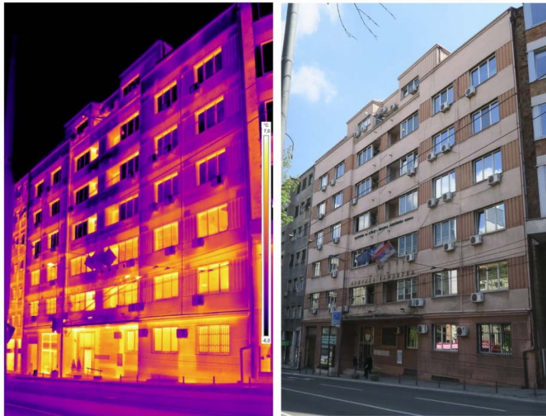
Figure 1. Thermal imaging and photograph of the street facade of the building of the City Municipality of Palilula. The image clearly shows heat losses in horizontal reinforced concrete cerclages as well as beams over windows. No vertical reinforced concrete elements are observed
