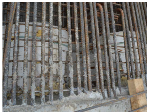
Figure 9. Deck slab reinforcement
