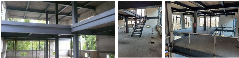
Figure 4. Steel construction of the upgraded part of the building / future library (Photo by author)
