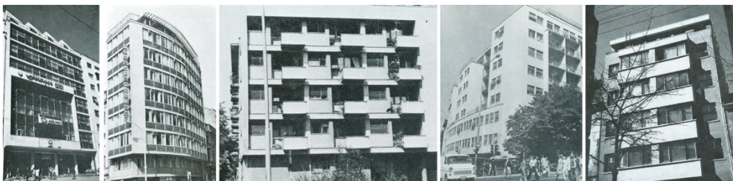
Figure 1. Architecture of Belgrade in the 6th decade of the 20th century (from left to right): 1-Business building, 1956, arch. A. Brkić, 2-Business building, 1958, arch. S. Mihailović, 3-Residential building, 1957, arch. D. Nastić, 4-Resid.-public building, 1958, arch. R. Bogojević, 5-Residential building, 1959, arch. Z. Petrović [1]
