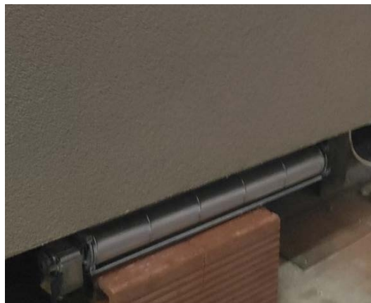
Figure 3. Cross flow fan under the PCM section.
