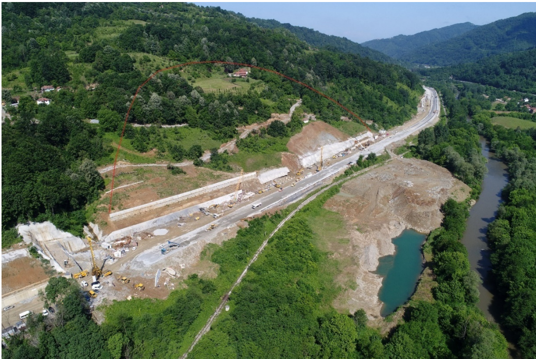
Figure 2. Formed landslide on the slope 2
