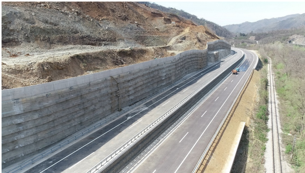
Figure 4. Formed landslide on the slope 1
