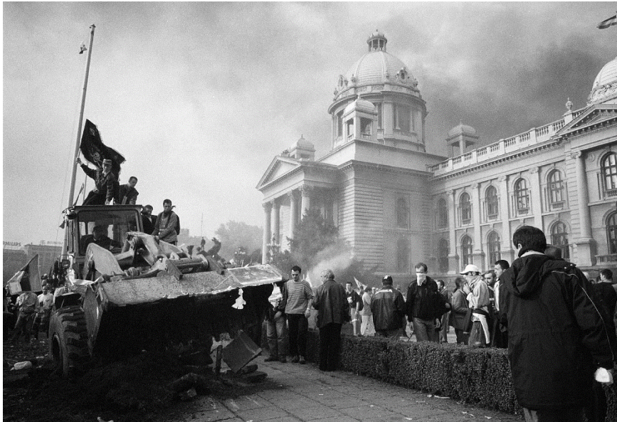
Figure 4. Bulldozer in front of the building
