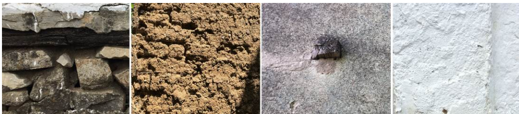
Figure 3. Photograph of used materials during construction of Petković family house in Laplje Selo
