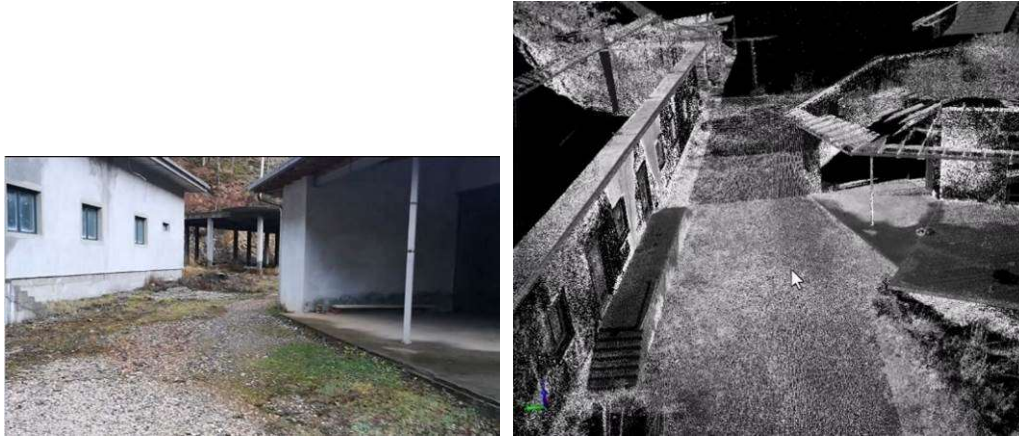
Figure 9. Actual situation (left), captured point cloud (right)
