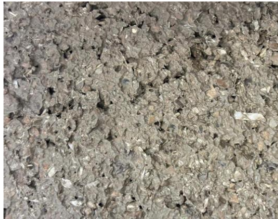
Figure 7. Compacted fresh concrete
