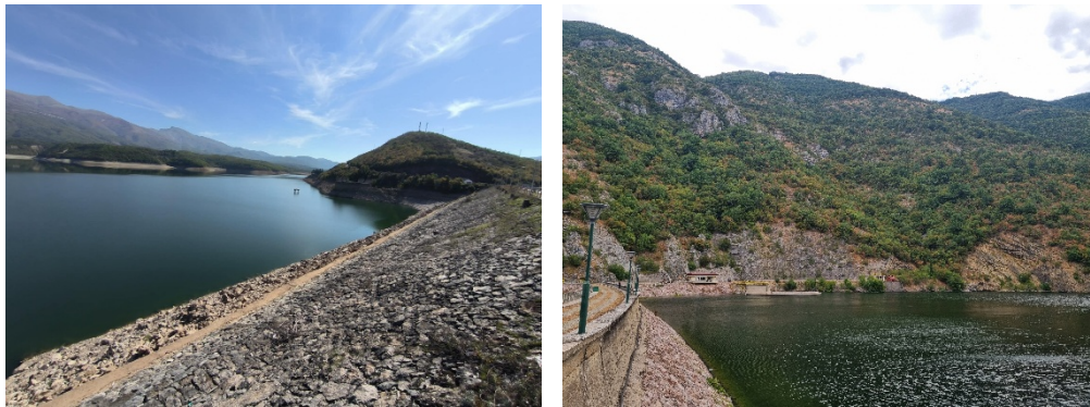
Figure 1. Shpilje Dam (left) & Globochica Dam (right) (photography by author).
