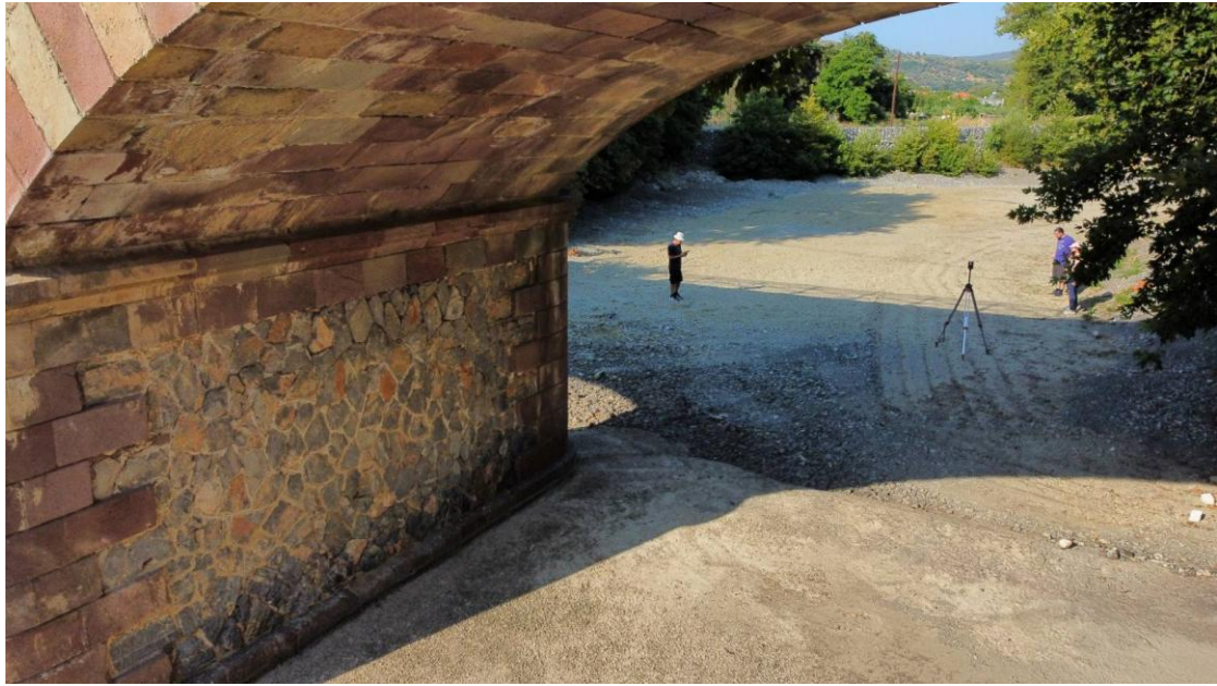
Figure 3. Terrestrial Laser Scanning workflow in an applied heritage context. The image illustrates the positioning of the BLK360 for generating TLS-derived point clouds of the Monodri Bridge's structural elements (Authors).
