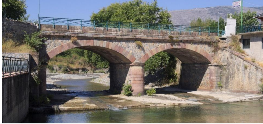
Figure 2. The Monodri Bridge, Evia, Greece. Detail of the two-arch stone structure highlighting the masonry and structural features of the arches [13].
