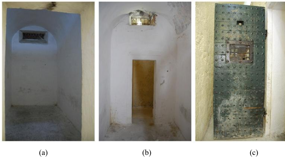
Figure 7. Typical Wing \Theta cell: (a) view from the entrance toward the interior, (b) view from the interior toward the entrance, and (c) detail of the cell door (Authors).
