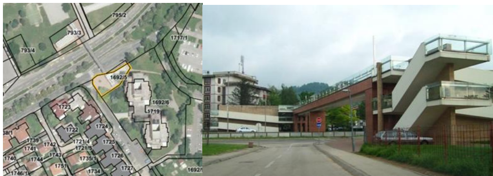
Figure 4. Pedestrian bridge in the city of Banja Luka (created by author).
