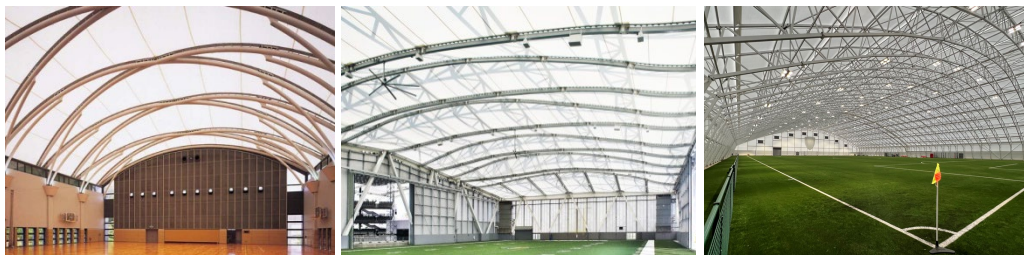
Figure 1. Example of tensile membrane structure used to cover large spaces [7], [8].
