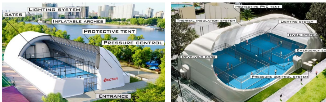
Figure 3. A new generation of double membrane systems with several innovative sustainable solutions [10].
