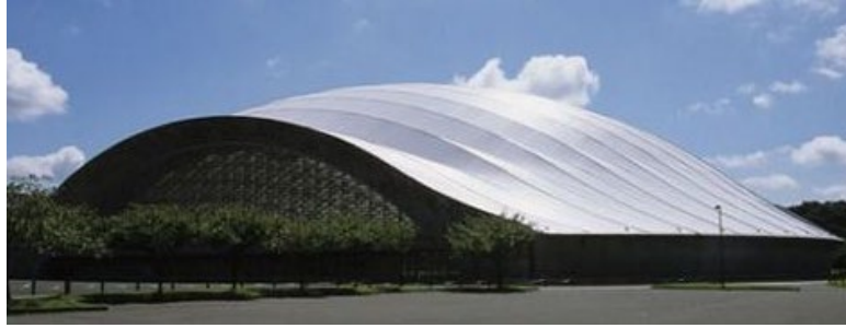
Figure 2. Frame-supported membrane structure, Akita Sky Dome in Japan [9].
