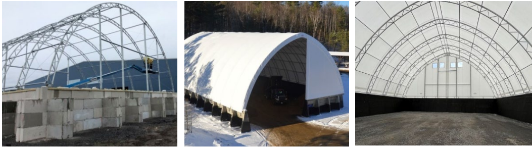
Figure 8. The integration of light membranes with robust, solid bases [13]
