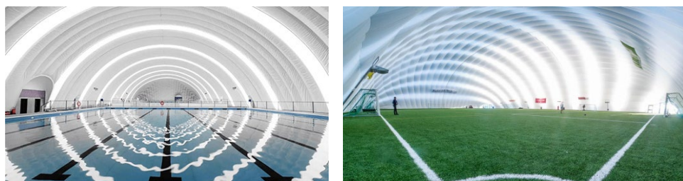
Figure 7. Air-supported membrane structures provides a space with a controlled environment [12].
