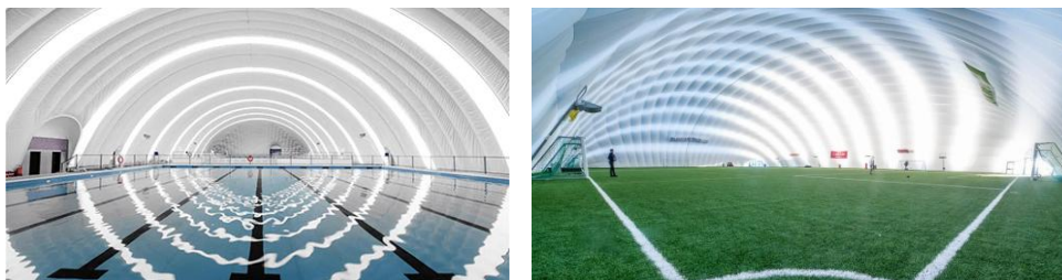
Figure 7. Air-supported membrane structures provides a space with a controlled environment [12].
