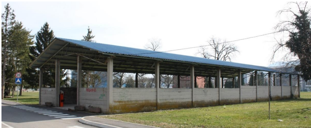
Figure 1. "Campus garage" at the University of Banja Luka (photography by author).
