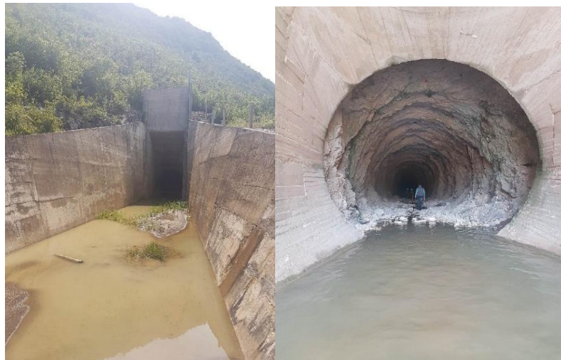
Figure 8. Entrance of the tunnel Dabarsko – Fatnicko polje (photography by author).
