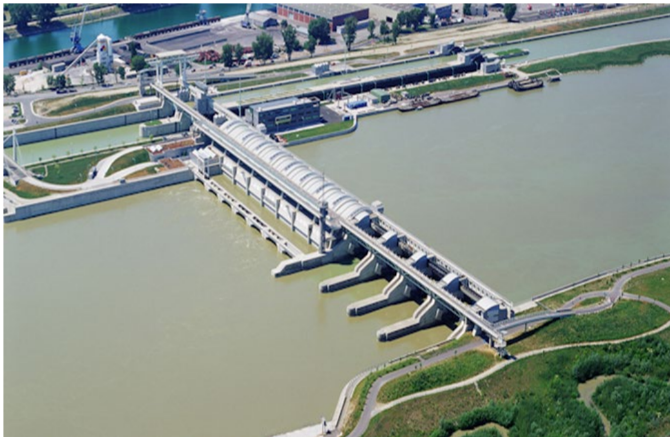
Figure 1. Aerial view of HPP Freudenu, showing the spatial relationship between the fish pass, the main Danube channel, and the “Neue Donau” diversion channel, provided as site context for the case study [9].
