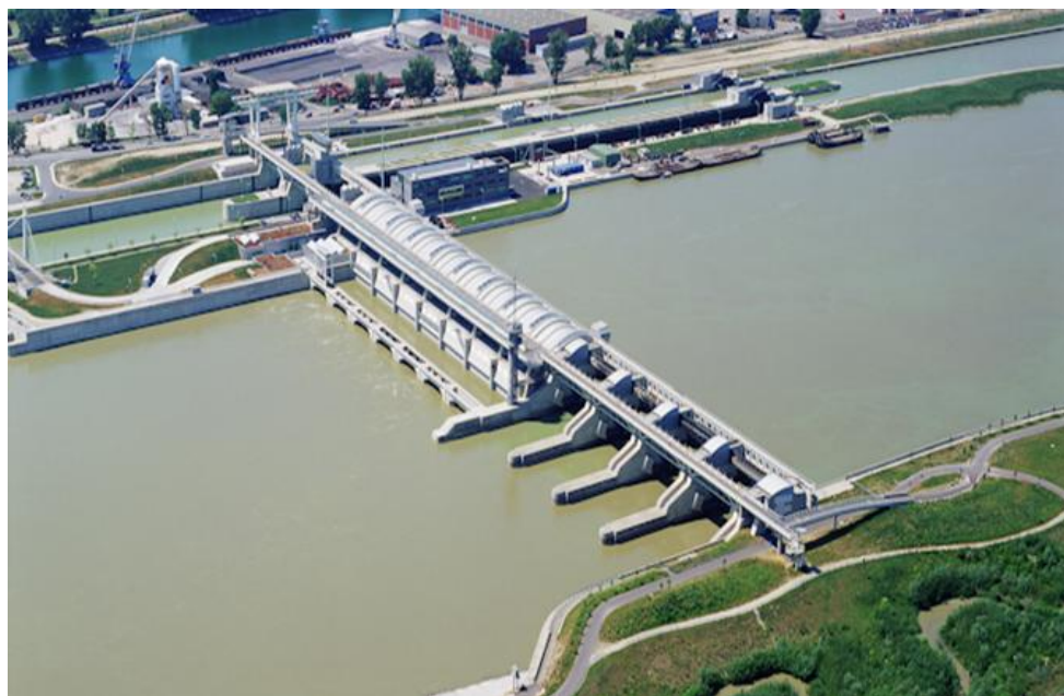
Figure 1. Aerial view of HPP Freudenu, showing the spatial relationship between the fish pass, the main Danube channel, and the “Neue Donau” diversion channel, provided as site context for the case study [9].
