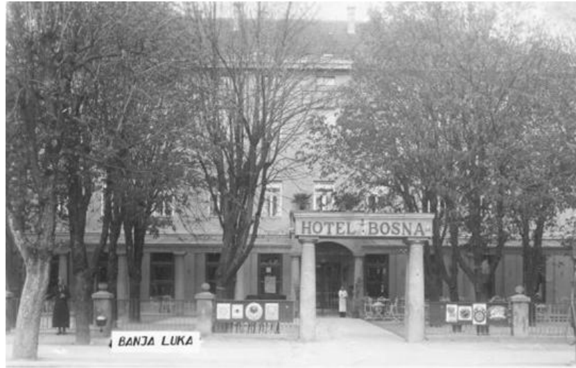
Figure 2. Hotel “Bosna”, entrance gate and lush vegetation, photographed after 1931. [8].
