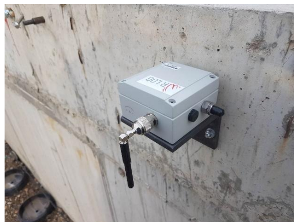
Figure 12. Tiltmeters installed on capping beams
