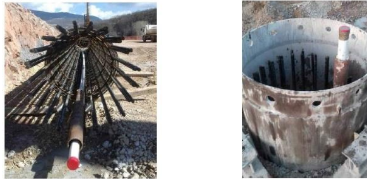
Figure 11. Inclinometers installed in piles (photography by author).
