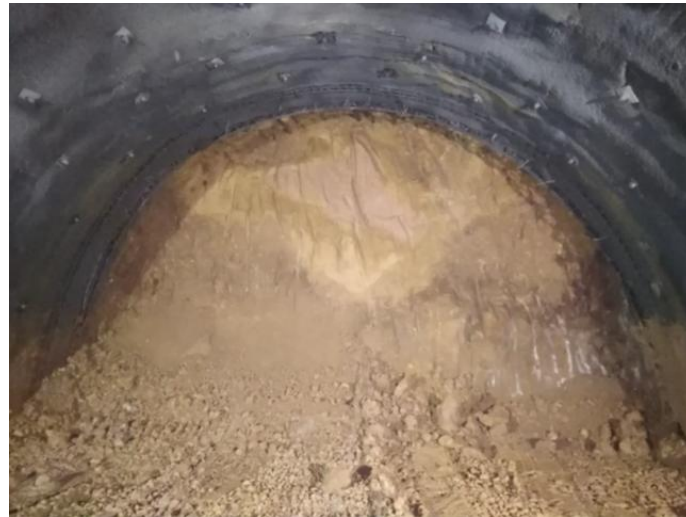
Figure 3. Tunnel face in glaciofluvial sediments, Ibarac tunnel (photography by author).
