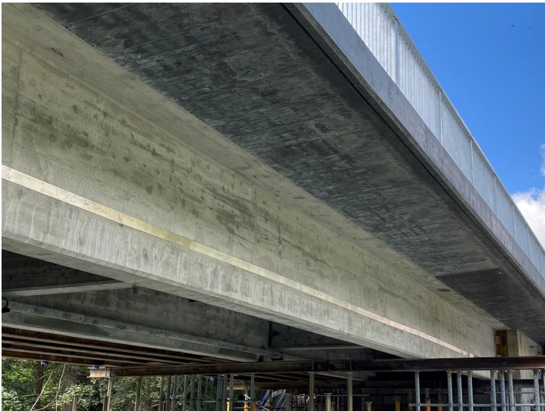
Figure 19. Existing girders in bright grey and UHFB cantilever slab in dark grey. Silver line represents an optical fiber for monitoring [21].
