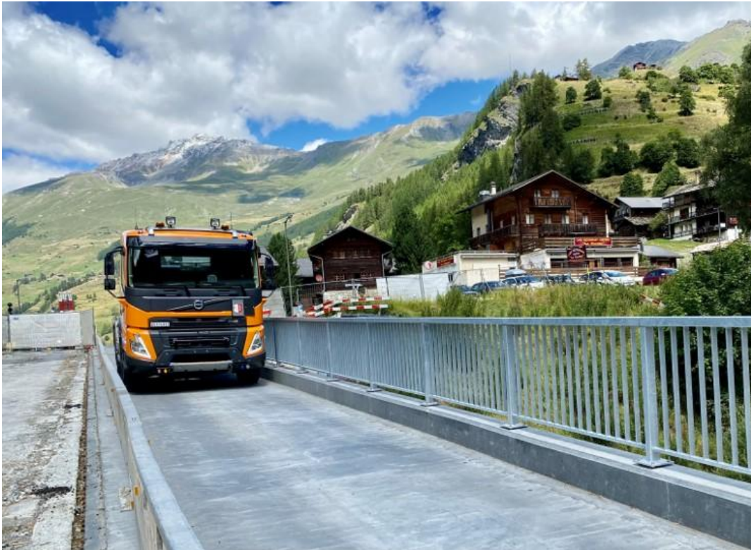
Figure 18. Phase 1 during construction period [21].
