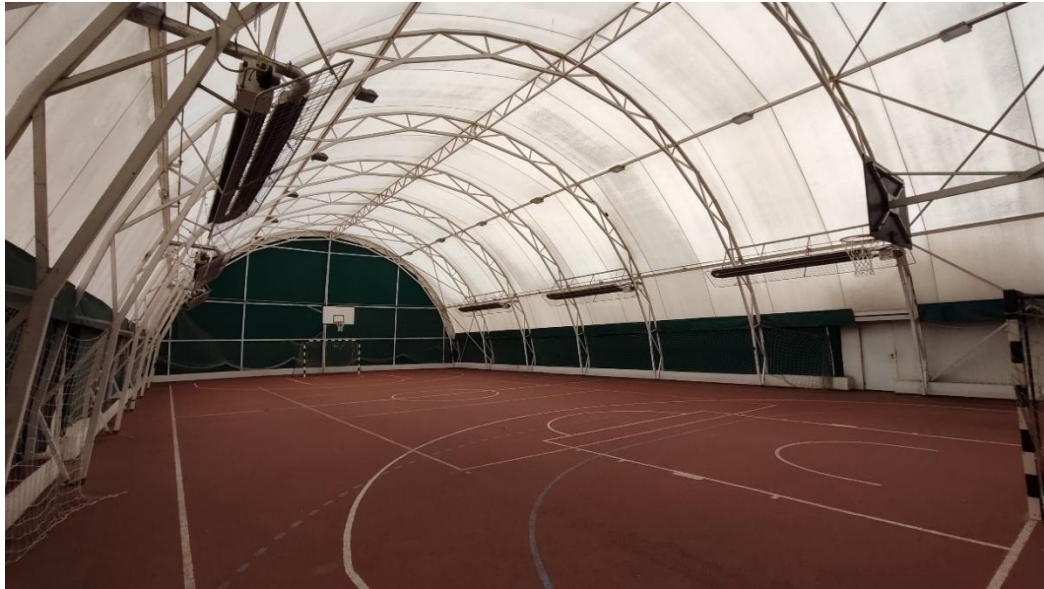
Figure 4. Interior view of the analyzed sports facility (source: photograph by authors).
