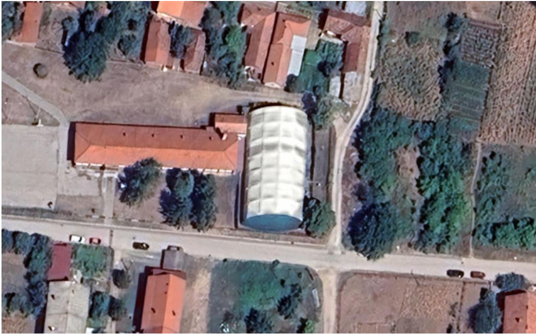
Figure 2. Near-by surroundings of the analyzed sports facility (source: Google Earth).
