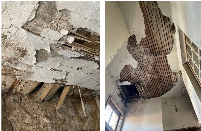
Figure 4. Current state of mezzanine construction (photography by author)
