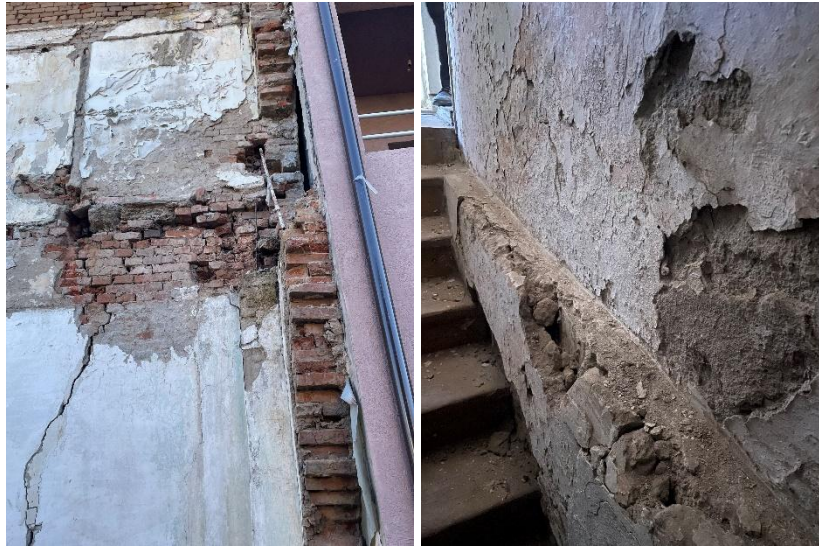
Figure 3. Current state of walls (photography by author)
