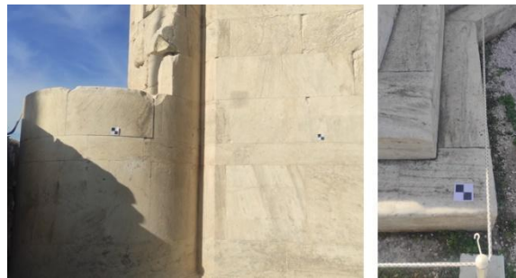
Figure 4. Figure 4. Checkerboard targets on the monument (photography by authors).
