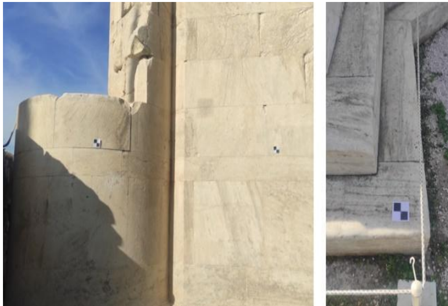
Figure 4. Checkerboard targets on the monument (photography by authors).
