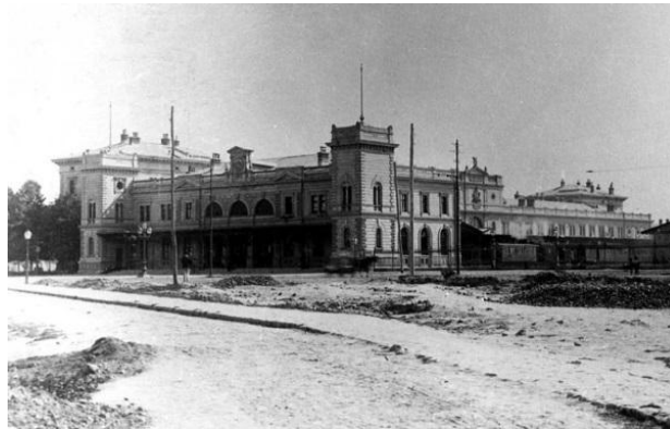
Figure 1. The appearance of Belgrade Railway Station after construction [9].
