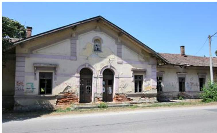
Figure 7. The present appearance of the Bela Crkva railway station [12].
