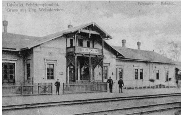
Figure 6. The former appearance of the Bela Crkva railway station [5].
