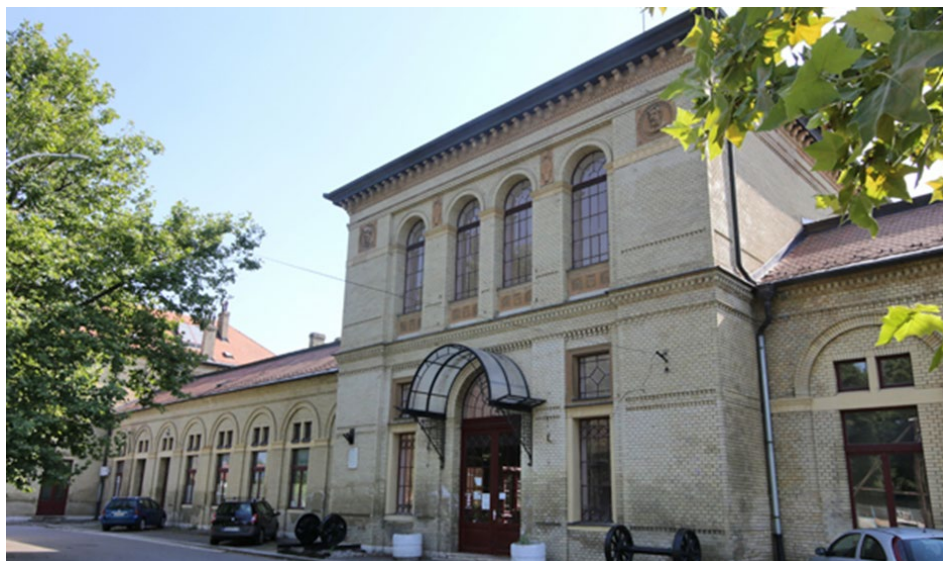
Figure 8. The present appearance of the Vršac railway station [13].
