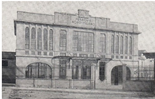
Figure 11. The former appearance of the Bullona railway station in Milan [22].
