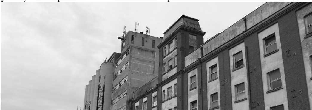
Figure 8. From right to left: The old Žitopek administrative building (a cultural good under previous protection), Square silo, and the 20 Žitopromet cylinder silos (photography by author).
