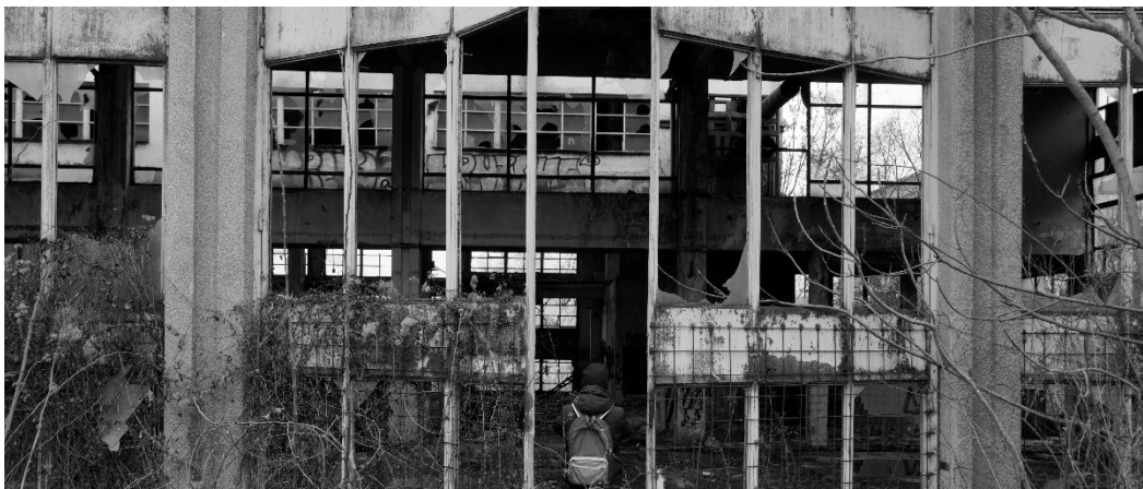
Figure 6. Entrance to an abandoned heating plant within the EI site (photography by author).
