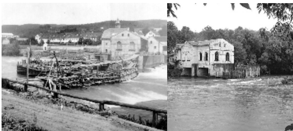
Photo 4, Construction of the power plant in Trapisti and its present condition / Source: Archive of the Urban Planning Institute of the Republic of Srpska, a.d., Banja Luka and photograph of the author /
