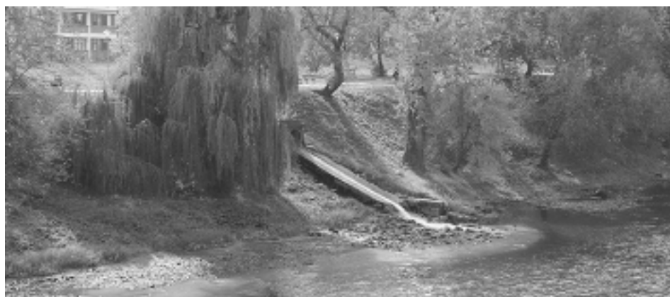
Photo 5 Banja Luka, park area in front of the University Complex downgraded by the sewage pipes / Source: Photo of the author /
