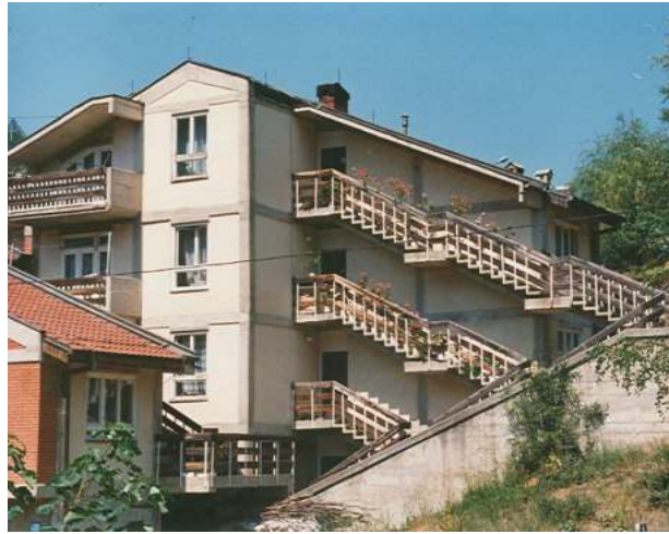
Figure 6. Multi-family residential building where each apartment has a separate entrance. Foreign experiences in the late 1970s in Crna Trava.
