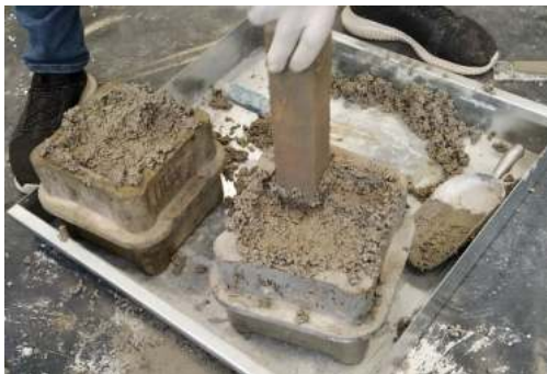
Figure 3. Casting of fresh concrete
