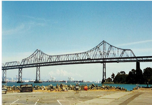
Figure 7. The appearance of the old East Crossing.
