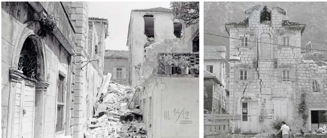
Figure 1. Markings on buildings after the 1979 earthquake classification indicating demolition or constructively rehabilitated
