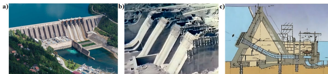
Figure 3. a) The Bajina Basta Dam, [14]; b) Construction of the Bajina Basta Dam, [15]; c) Cross-section of the Bajina Basta Dam, [16].
