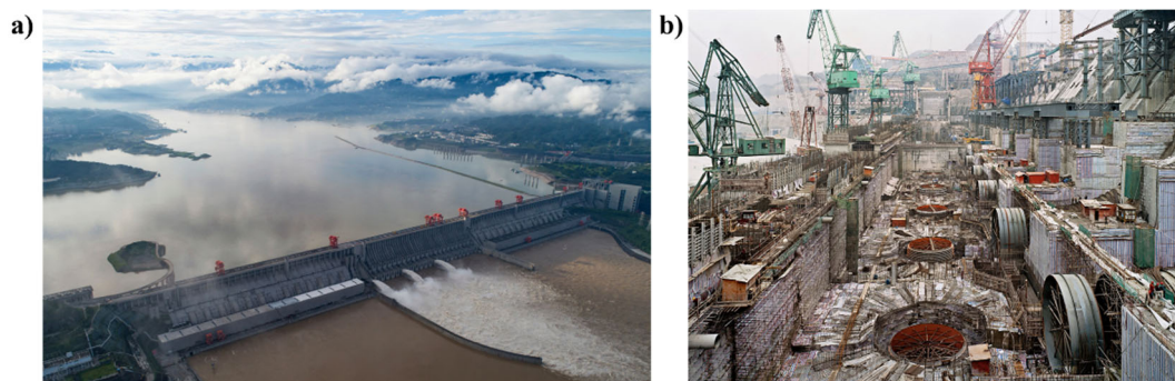
Figure 8. a) Three Gorges Dam, [30]; b) Construction of Three Gorges Dam, [31].
