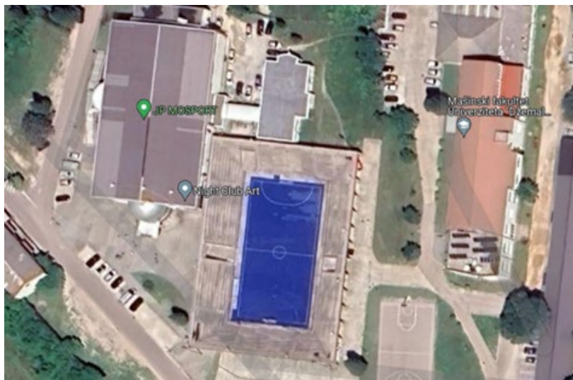
Figure 1. Aerial view of the stadium structure
