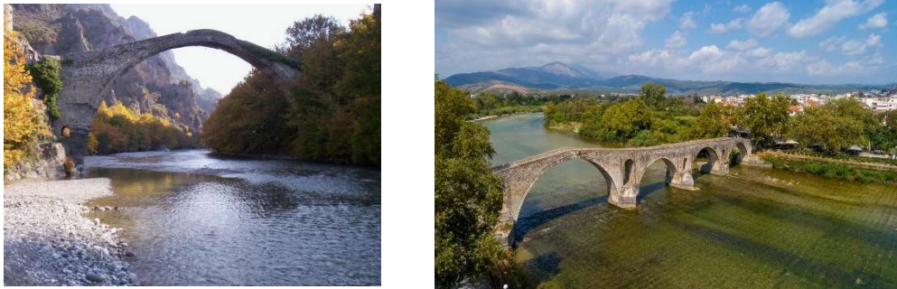
Figure 1. a) The single-arched stone bridge of Konitsa ( https://www.allovergreece.com ) b) The multi-arched stone bridge of Arta ( https://discoverarta.gr/ )
