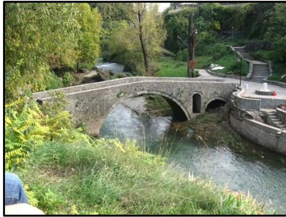
Figure 3. View of the bridge (authors, 2022)
