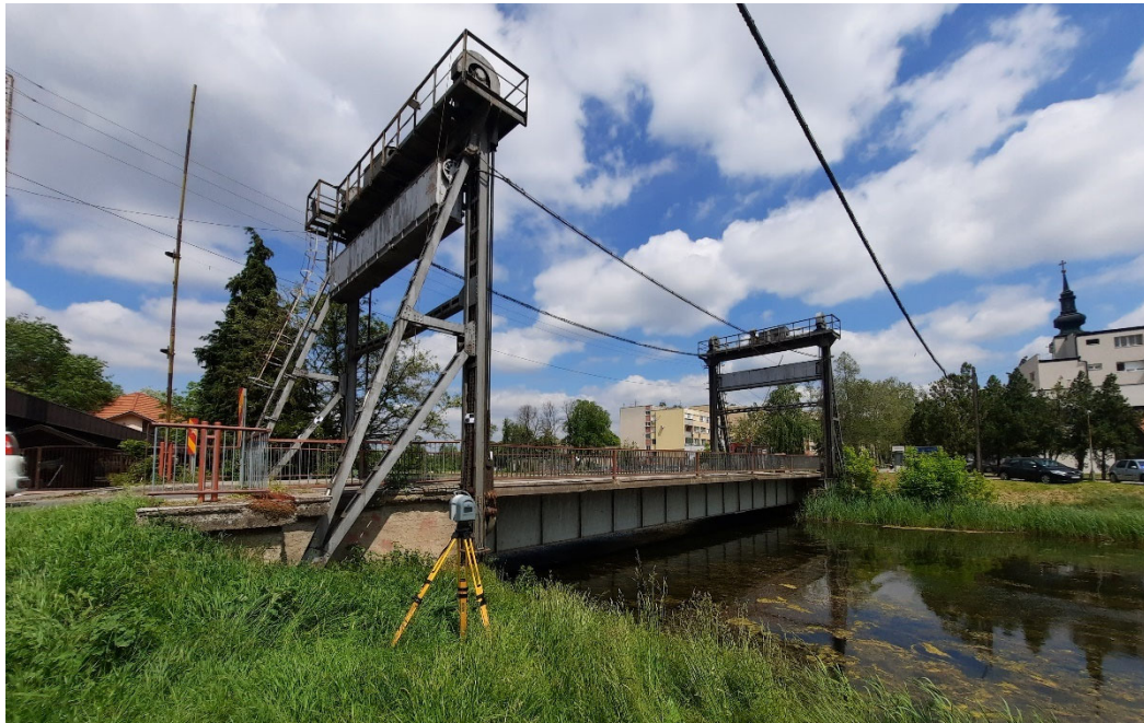
Figure 3. Bridge in Kula, scanner position 1.
