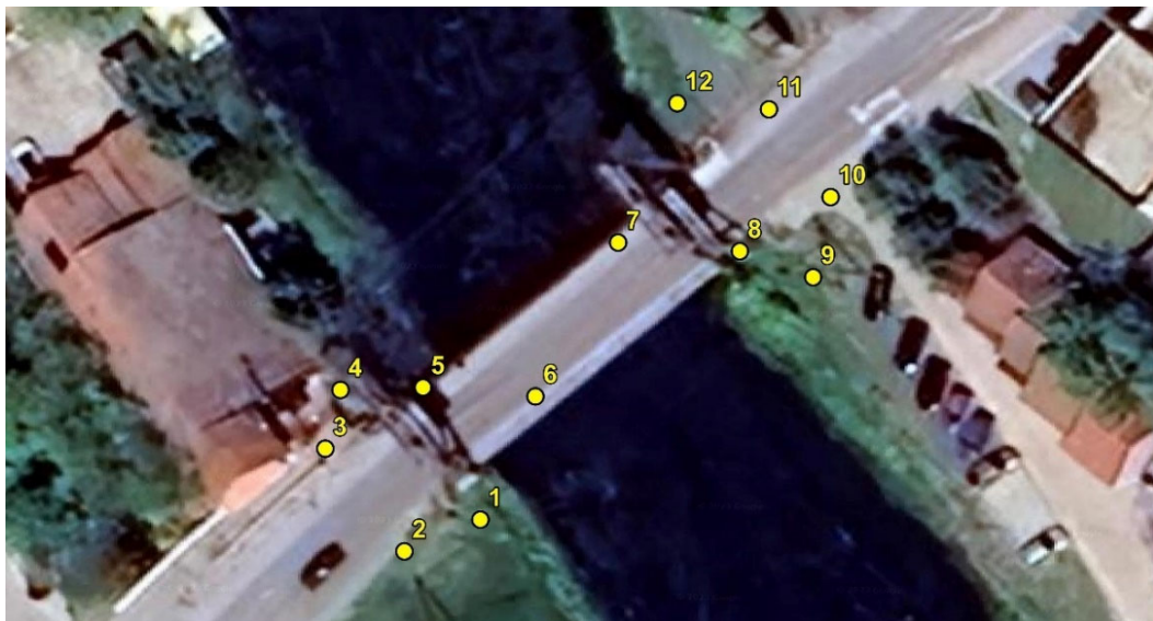
Figure 2. Scanner positions during terrestrial laser scanning of the bridge.
